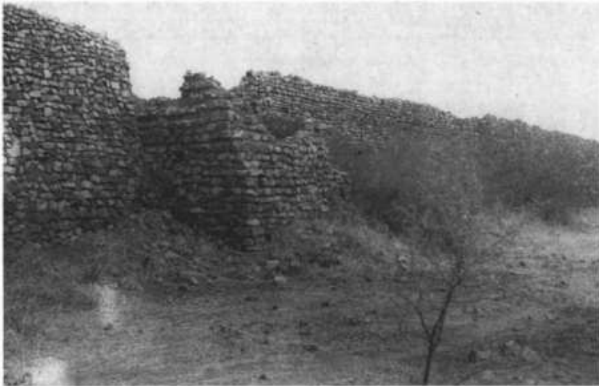
PLATE 23.2 Ruins of a defensive tower of the tata (fortress) at Hamdallahi
